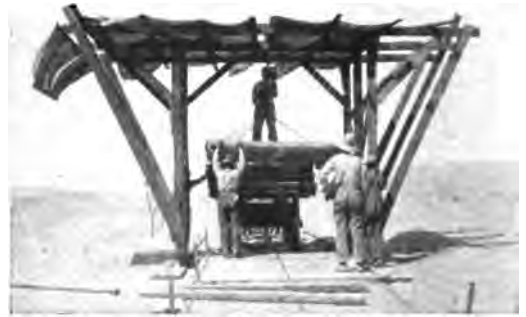
PLACING A SECTION OF THE PORTABLE ROAD
